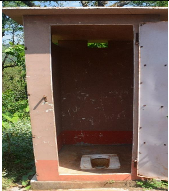
Bathrooms built with durable materials, easy to clean, with ventilation, lighting, and a door with a closing mechanism.
