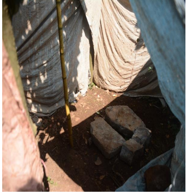
Latrine without a door, and with a flooded floor without drainage, and without a door that guarantees the privacy and security of those who use it.
